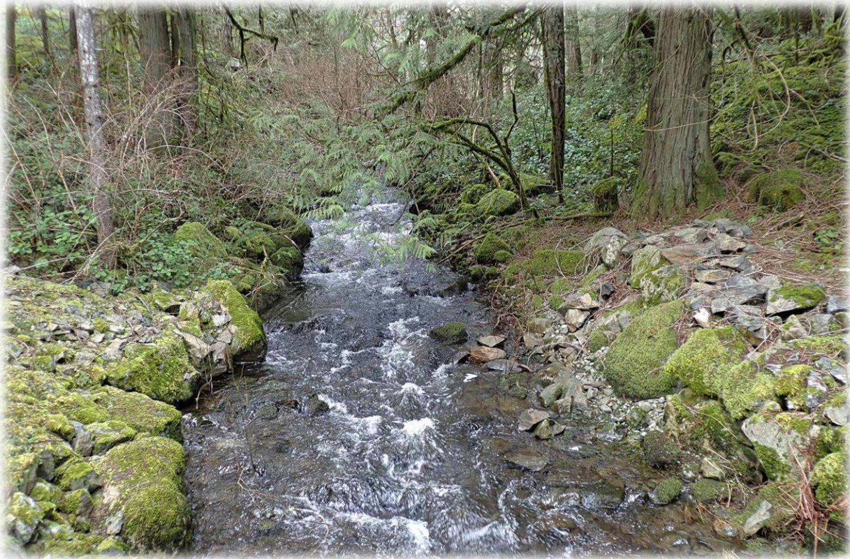
Figure 5. Millstream Creek flows through a culvert beneath the paved road south of Polygon 24
